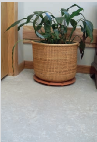
Photo 1: Flaw or feature? Equinox House has an unsealed concrete floor at present while analyses of thermal energy and moisture flows are being studied. Figure 1: "Coast" inside ambient air temperature data collected from the old Newell house, the Washburne Trade School passive solar house and Equinox House. Note that the "stairsteps" in the old Newell house data is due to an old 8-bit data acquisition system.
