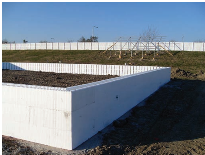
Photo 1 (left): Installation of the insulated concrete form (ICF) foundation blocks around Equinox House perimeter. Note the plastic web that both holds the Styrofoam walls together and supports the rebar. Photo 2 (right): ICF foundation wall prior to pouring concrete. Note that the concrete footer below the ICF wall is close to the original grade of the surrounding ground.
