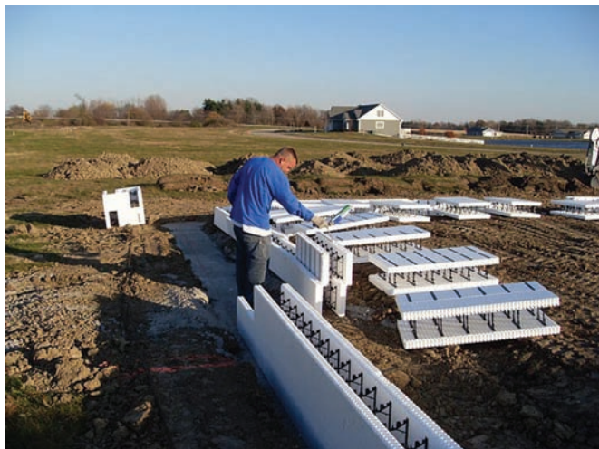
Photo 1 (left): Installation of the insulated concrete form (ICF) foundation blocks around Equinox House perimeter. Note the plastic web that both holds the Styrofoam walls together and supports the rebar. Photo 2 (right): ICF foundation wall prior to pouring concrete. Note that the concrete footer below the ICF wall is close to the original grade of the surrounding ground.
