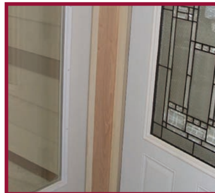
Photo 2: 12 in. (300 mm) thick walls allow for two full size doors to improve air sealing and insulation value.
