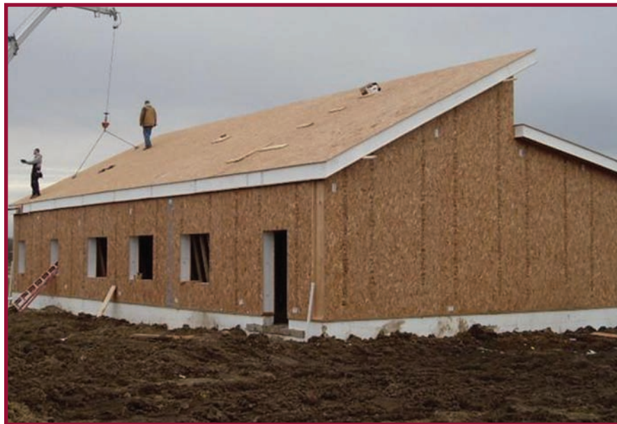
Photo 1: Equinox shell consisting of 12 in. (300 mm) thick wall and roof SIPs.
