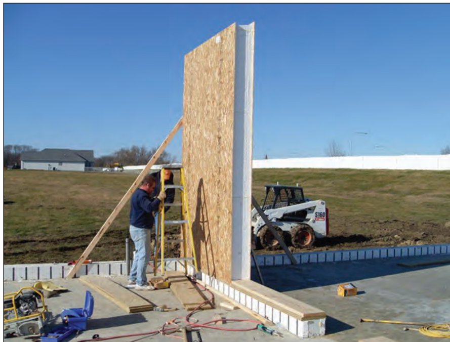
Photo 1: Installation of the first structural insulation panel.
