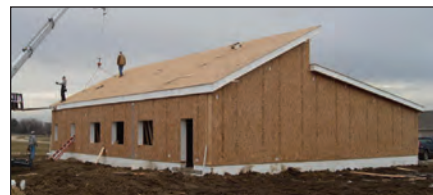
Photo 2: Installing the last SIP on the roof.
