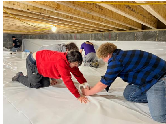
Figure 4 Students working to tape and seal poly sheeting.
