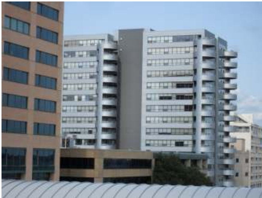
South side of an overglassed building. Based on the shades drawn, 15 percent of the windows used would have been sufficient, resulting in less cost, less energy, and more comfortable occupants.
