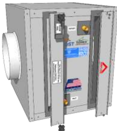
Reverse access panels and reinstall nuts. Note: Airflow Sticker should now point Left-to-Right.
