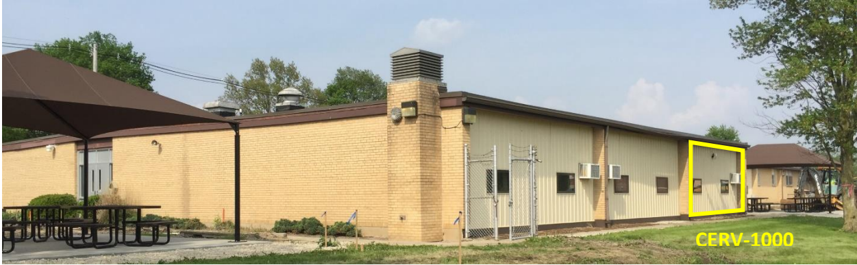
Figure 2 Three of 12 classrooms on the southwest side of Georgetown-Ridge Farm school district's Mary Miller Junior High School. Highlighted is CERV-1000 Unit#1's classroom location.
