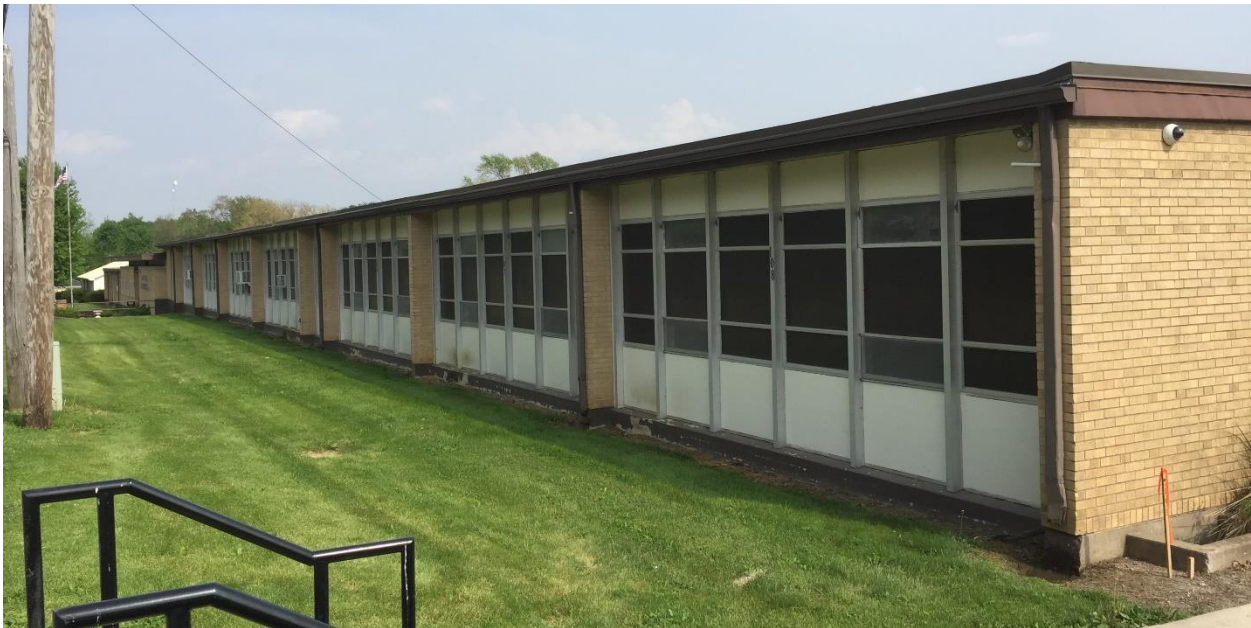
Figure 3 Outdoor heat pump units and electrical disconnects can be installed on these 6 classrooms on the north side of MMJH School and on 5 classrooms on the south side anytime G-RF facilities staff schedule allows while awaiting delivery of the next 11 CERV-1000 units. CERV-1000 units can be set in place in their classrooms while awaiting installation scheduling that avoids classroom disruption.
