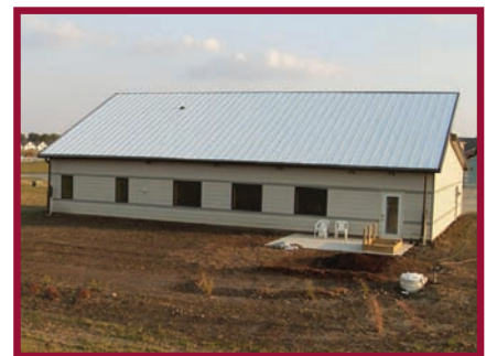
Photo 3: North looking view of Equinox showing the main living space picture windows and smaller casement windows in the master bedroom. Note the 1,700 gallon (6435 L) cistern access cover for rainwater harvesting and adjacent rain garden area for storm water retention in the foreground.
