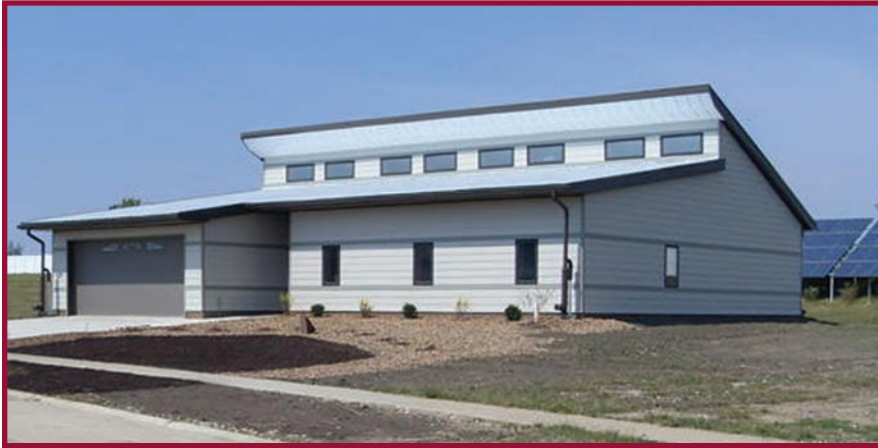
Photo 1: Equinox House near the fall equinox (September 20) with clerestory overhang and lower roof overhang allowing full sun to enter the house.
