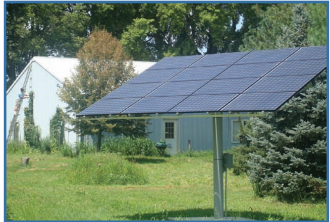
Photo 1: Snow covered solar array at Equinox House in December 2010 at sunrise. Note the “solstice” stone in the foreground with its shadow marking the sunrise solar azimuth angle. Photo 2: Our laboratory’s 3.2 kW, two-axis tracking array was installed in July 2008. Note Ben on ladder harvesting hops planted along the south wall of the lab for shade. The light colored wall behind the hops is 10°C (18°F) cooler than unshaded wall regions during sunny summer days.
