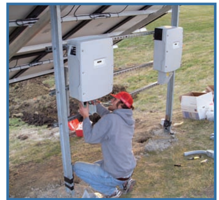
Photo 3: Installation of one of the twin 6 kW solar PV system inverters for the Equinox House solar system.
