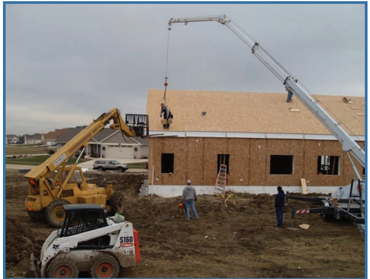
Photo 4: View of the mini-front end loader, forklift and crane used during house panel erection. Other site equipment used for construction are the backhoe and mini-excavator.
