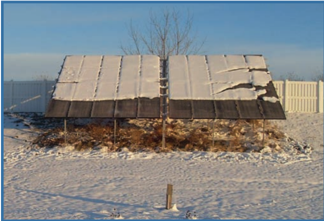
Photo 1: Snow covered solar array at Equinox House in December 2010 at sunrise. Note the “solstice” stone in the foreground with its shadow marking the sunrise solar azimuth angle. Photo 2: Our laboratory’s 3.2 kW, two-axis tracking array was installed in July 2008. Note Ben on ladder harvesting hops planted along the south wall of the lab for shade. The light colored wall behind the hops is 10°C (18°F) cooler than unshaded wall regions during sunny summer days.
